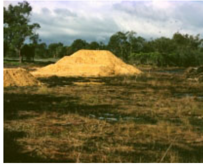
Load testing sand, heaps of clearing in foreground - destruction of samphire. Jul.'95.
