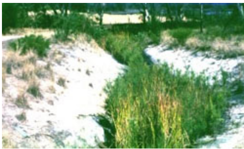
Open Section of Drain for Run-off Water of Subdivision.
